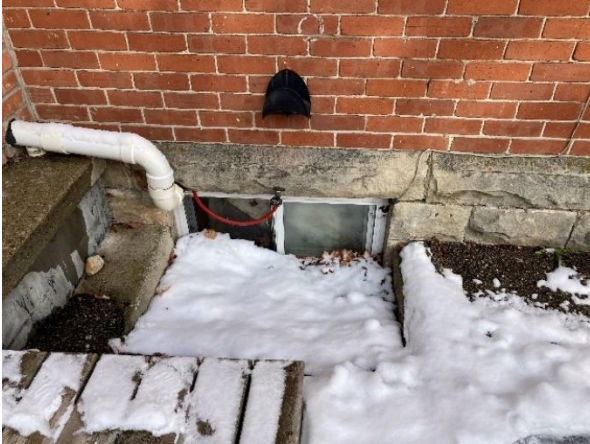
Plate 21: Cut stone foundation
