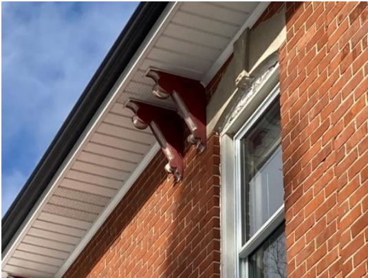
Plate 19: Overhanging eaves and paired bracket detail
