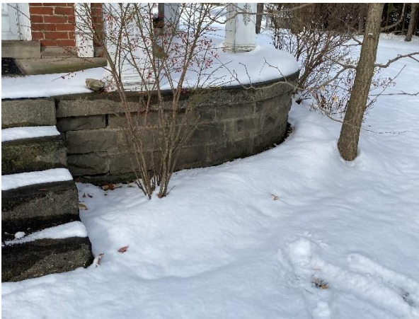
Plate 27: Stone foundation of the front and side porches
