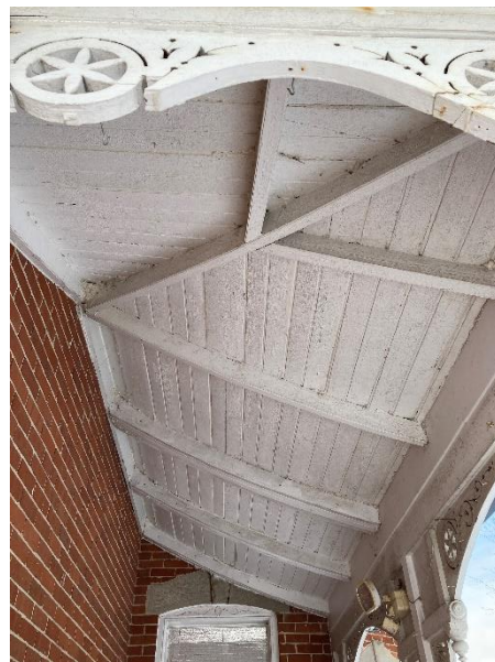
Plate 28: Bellcast roof of the side porch
